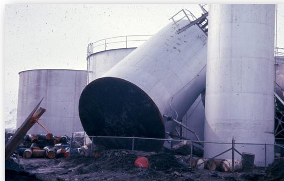
*Structural damage and ground failure during the 1964 Great Alaska Earthquake: Cover – residence in the Turnagain Slide, Anchorage; Above – overturned fuel tank at the Port of Anchorage.*
