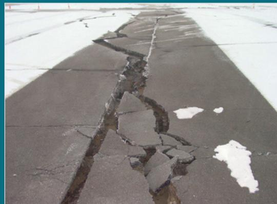
**FIGURE 2:** Ground failure in the Northway Airport runway, 2002 Denali Earthquake
