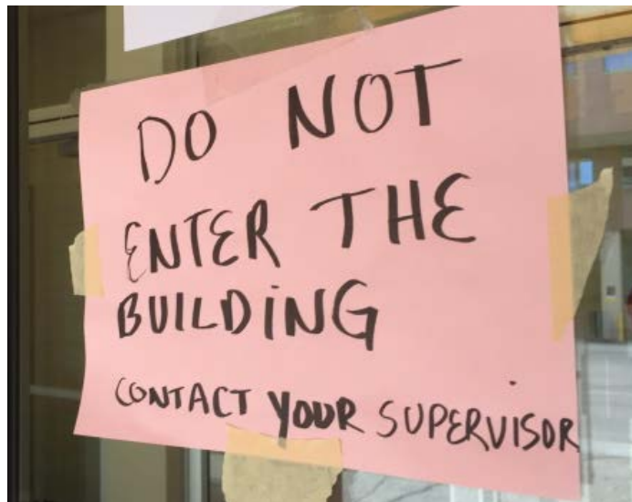
Shaking damaged the Yukon government's Lynn Building in Whitehorse, necessitating its closure until it could be inspected for safety. (Photo credit: Philippe Morin/CBC)
