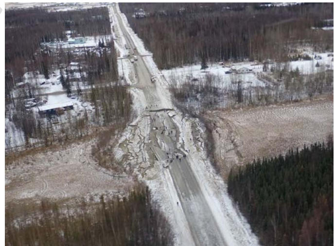
Lateral spreading disrupted Vine Road near Wasilla. Many failures of engineered materials occurred on or adjacent to water-saturated lowlands. (Photo credit: U.S. Geological Survey)
