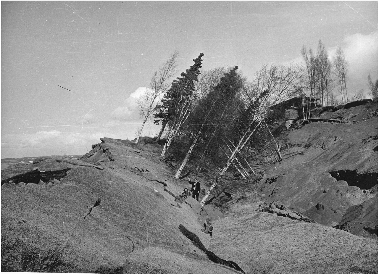
Turnagain Heights slide, Anchorage, 1964
